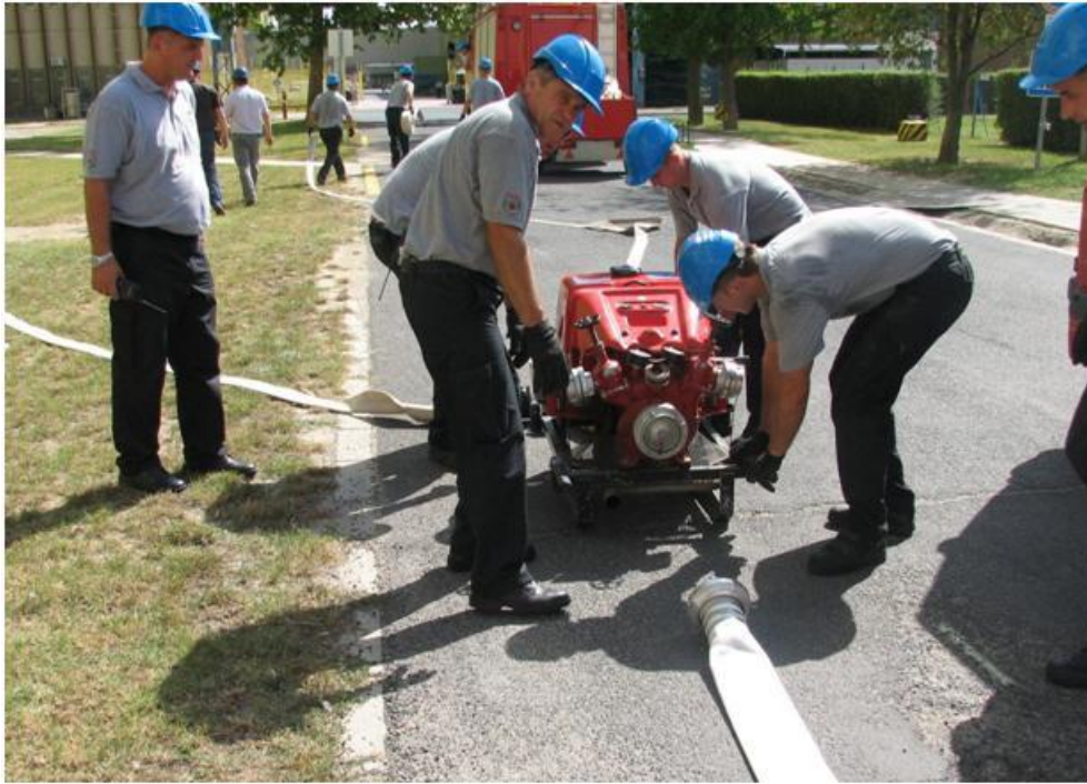
Figure 5-1: Installation of the mobile water supply system
