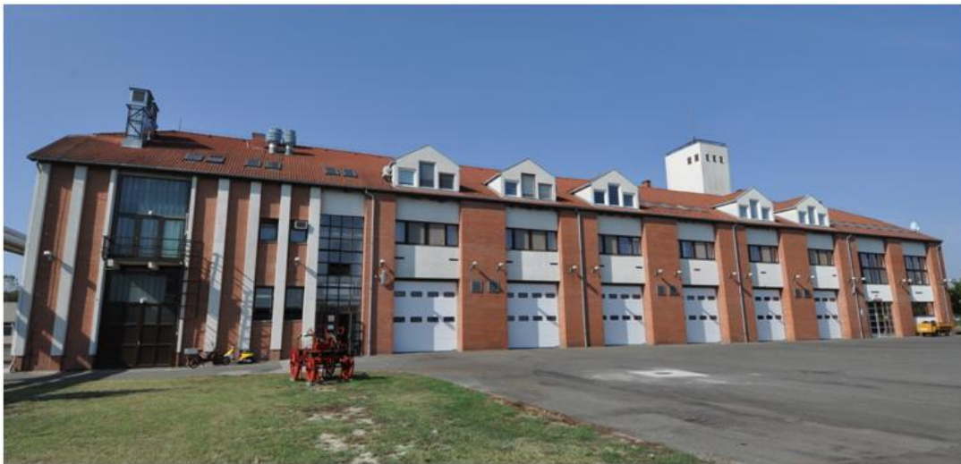
Figure 2-6: Fire brigade barrack on the NPP site
