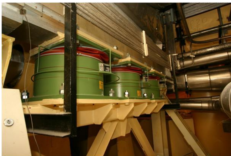
Figure 2-4: Reinforcement by viscous snubbers
